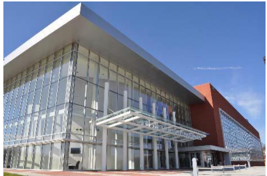
The JSNN Building at Gateway University Research Park.
